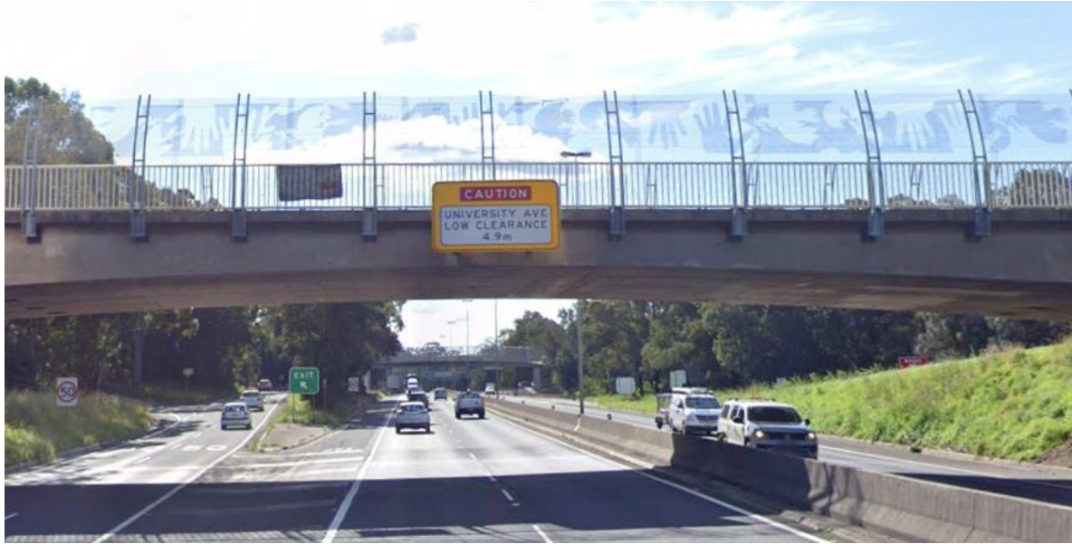
Figure 2.4: Height restriction - University Avenue footbridge, Gwynneville
