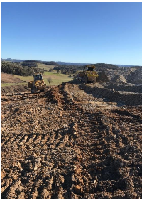
Earthworks begin on wind farm
