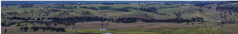
Crookwell 3 Wind Farm Site
