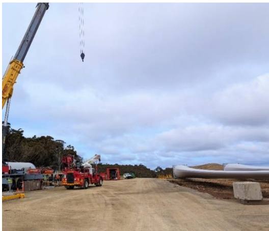
Crane laying down the blades next to the foundation
