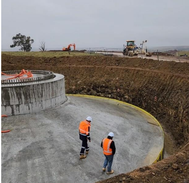
GPG Site manager, Borja, inspecting the last foundation poured
