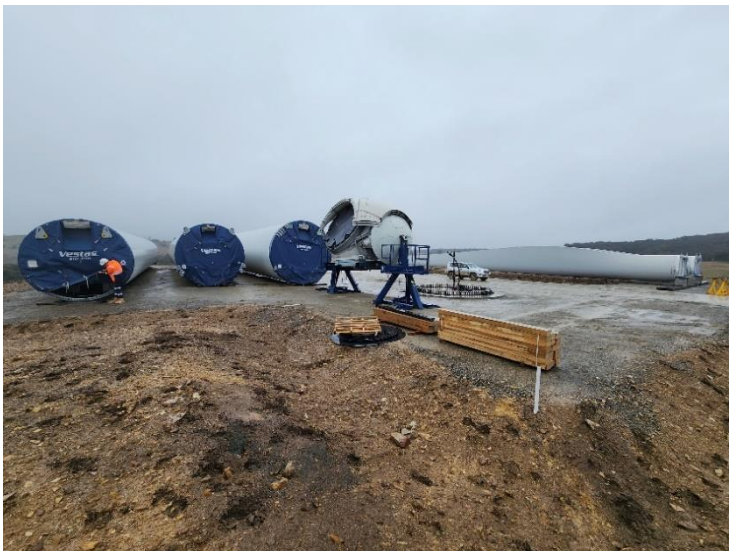
Components of a turbine at Crookwell 3 Wind Farm
