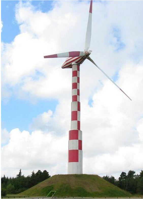
Tvindkraft, the world's first multi- megawatt wind turbine was built near Tvind in 1978
