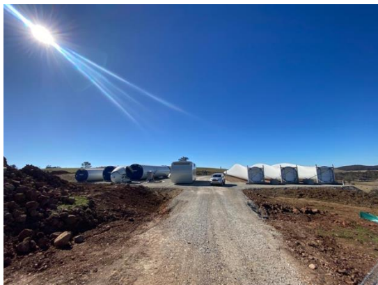
Components laying down, next to the foundations.
