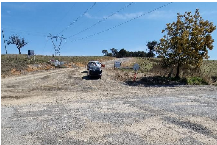
Trenching and cabling on Woodhouselee Rd. completed.
