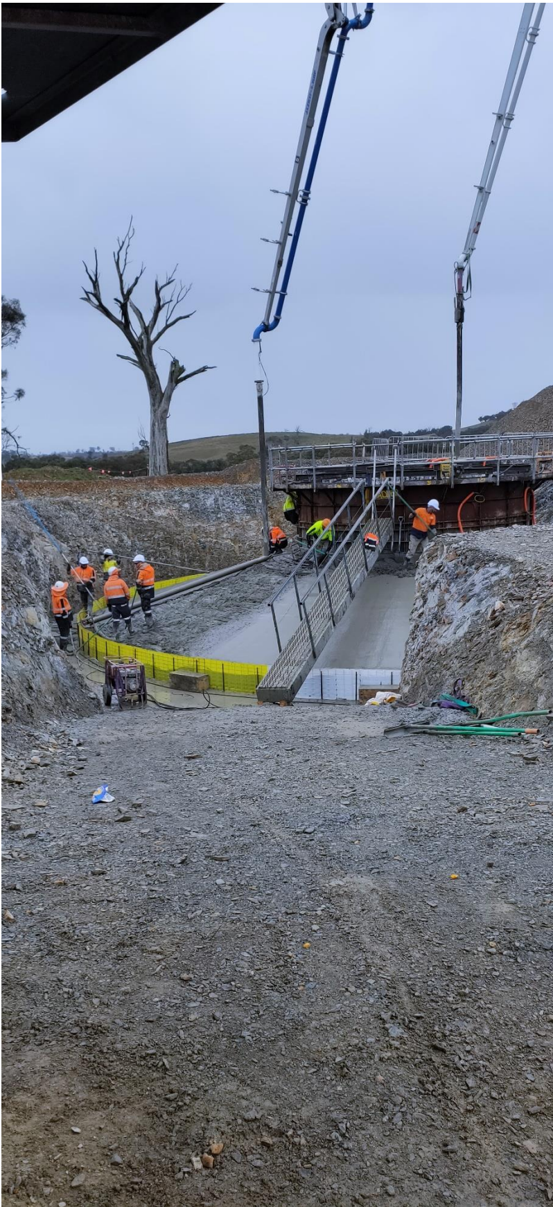
Photograph 12 - Concrete pour for the footings of a Wind Turbine
