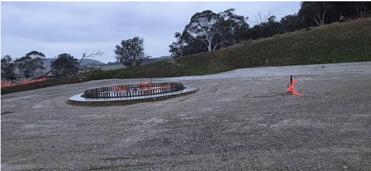
Photograph 4 – Footing of a completed Wind Turbine and pad area
