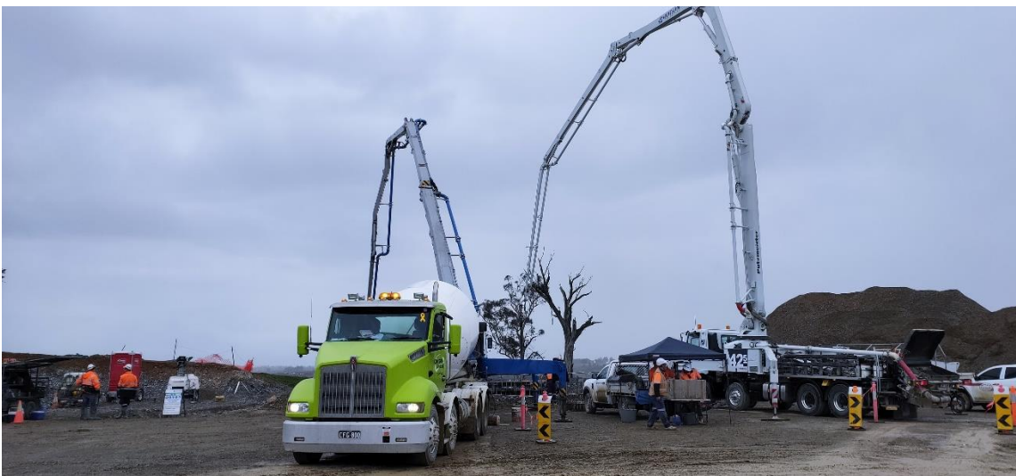
Photograph 11 - Pouring the footings for Wind Turbine
