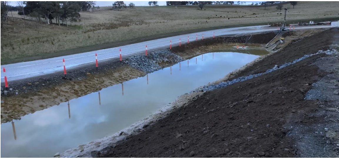
Photograph 10 - Sediment basin at concrete batch plant
