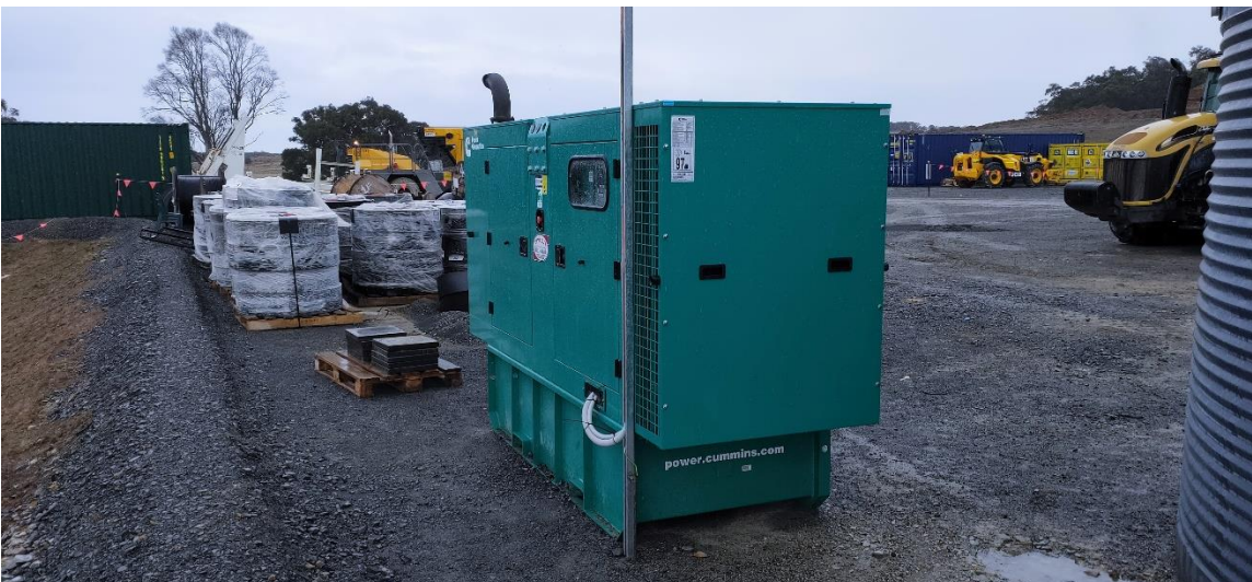
Photograph 9 – Laydown yard clearly delineated and site generator is self bunded
